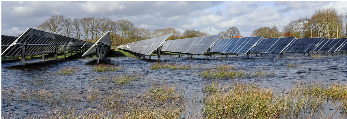
Wattmanufactur - Solarpark Lottorf ( https://wattmanufactur.de/moor-pv.html )
